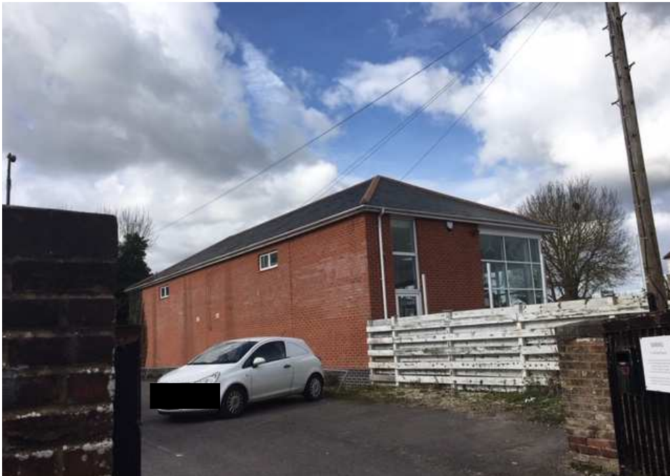
View of building south west of site from Station Road
